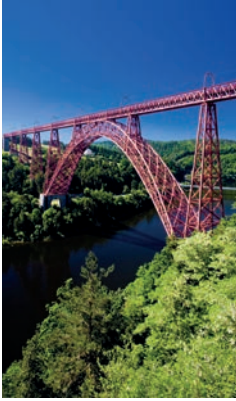
Garabit Viaduct, France.
