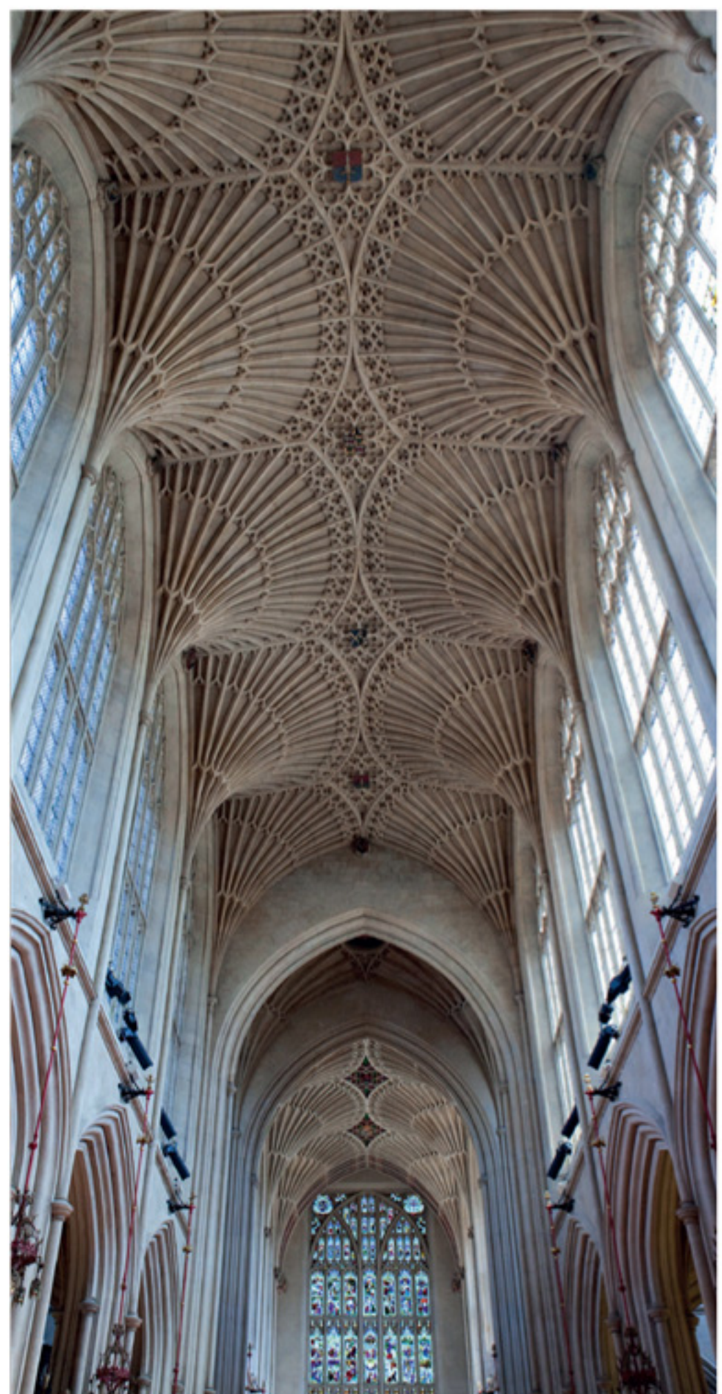
Intricate fan vaulting inside Bath Abbey.
